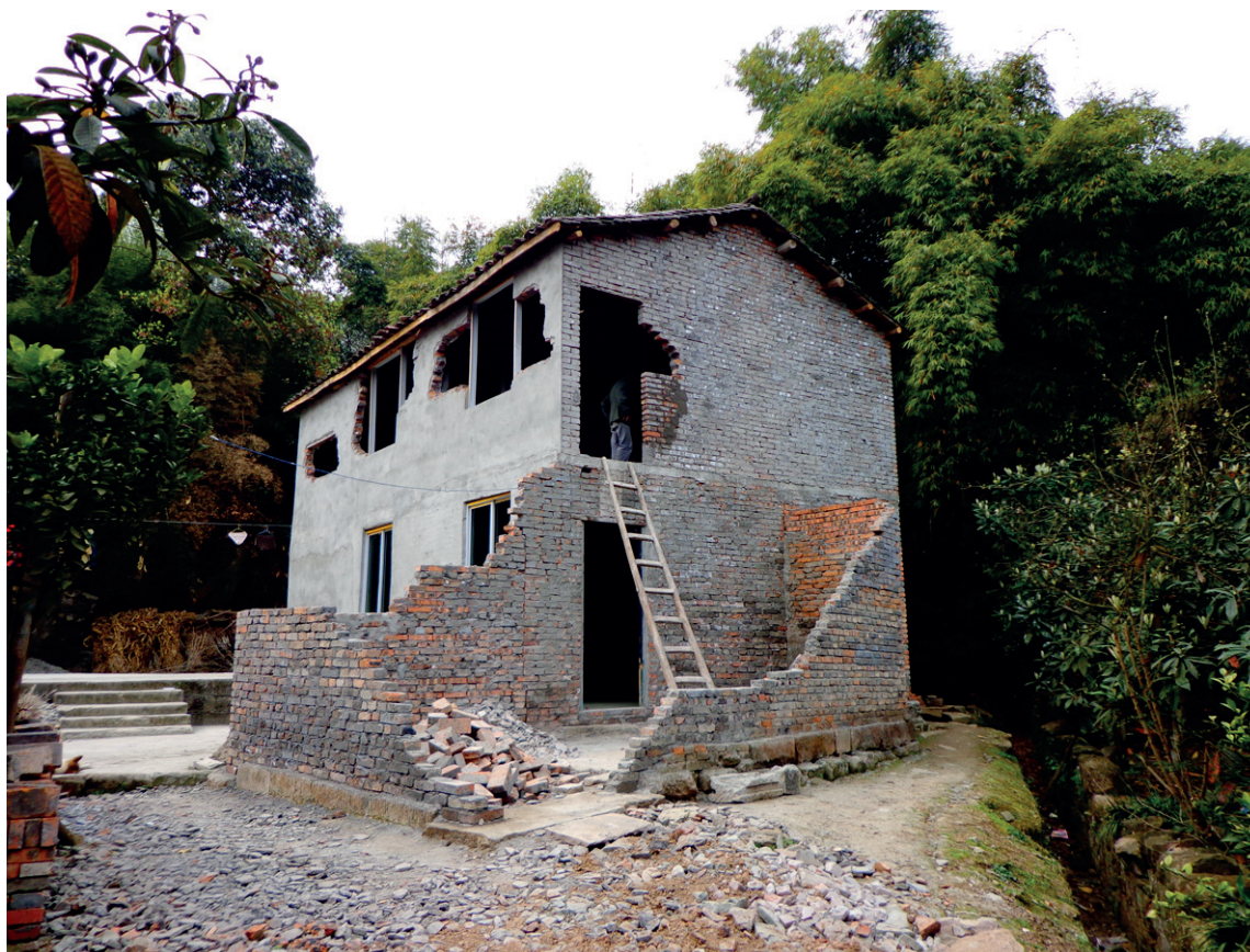
Fig. 1. A recently renovated building which has been repeatedly damaged by staff from the township's demolition office.
